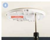
Attach base to ceiling with screws.
