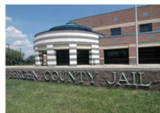
Bergen County Jail 820 MOBOTIX Cameras, U.S.A.
