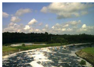
S. Florida Water Management District 147 MOBOTIX Cameras, U.S.A.
