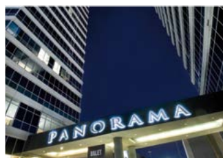
Panorama Towers 137 MOBOTIX Cameras, U.S.A.
